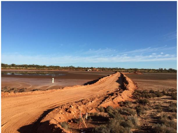
Figure 2: On-playa causeway developed to assess geotechnical properties of borrow material
