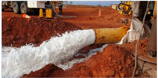
Figure 3: 19LWPR002 being developed into the southern strike of the Lake Wells palaeochannel has been cased to a depth of 175.5m (previous deepest well cased to 170m) and is indicating very high flow rates
