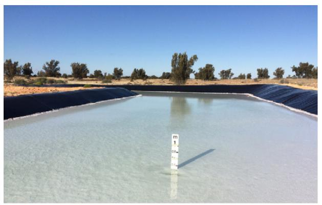
Figure 1: Pre-concentration pond at the Lake Wells SOP project prior to initial brine transfer
