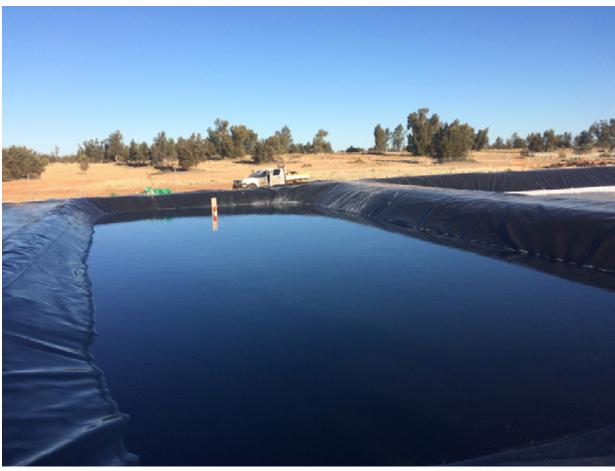
Figure 2: Pre-concentrated brine after transfer into harvest pond 1
