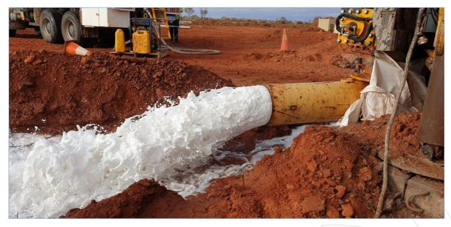
Figure 1: 19LWPR002 being developed into the southern strike of the Lake Wells palaeochannel has been cased to a depth of 175.5m (previous deepest well cased to 170m) and is indicating very high flow rates
