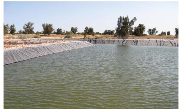
Figure 2. Pilot Solar Evaporation Pond at Lake Wells
