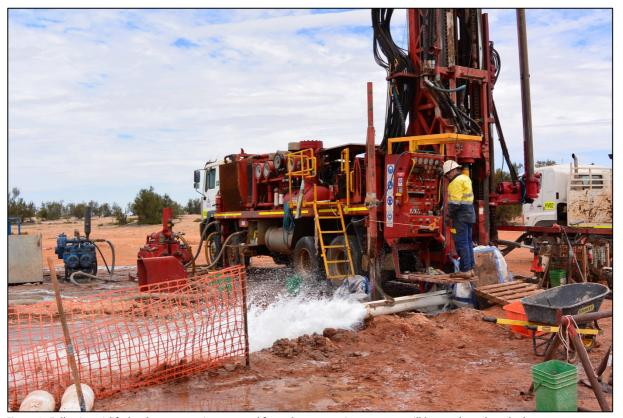
Figure 2: Following airlift development, a rigorous and formal test-pumping program will be conducted on the bores
