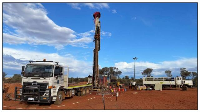
Figure 4: Drill rigs have been mobilised to site preparing and developing the Western Borefield
