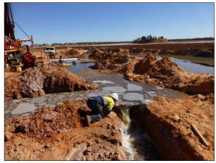
Figure 4: Airlift development of test-production bore #2 Site A with v-notch testing
