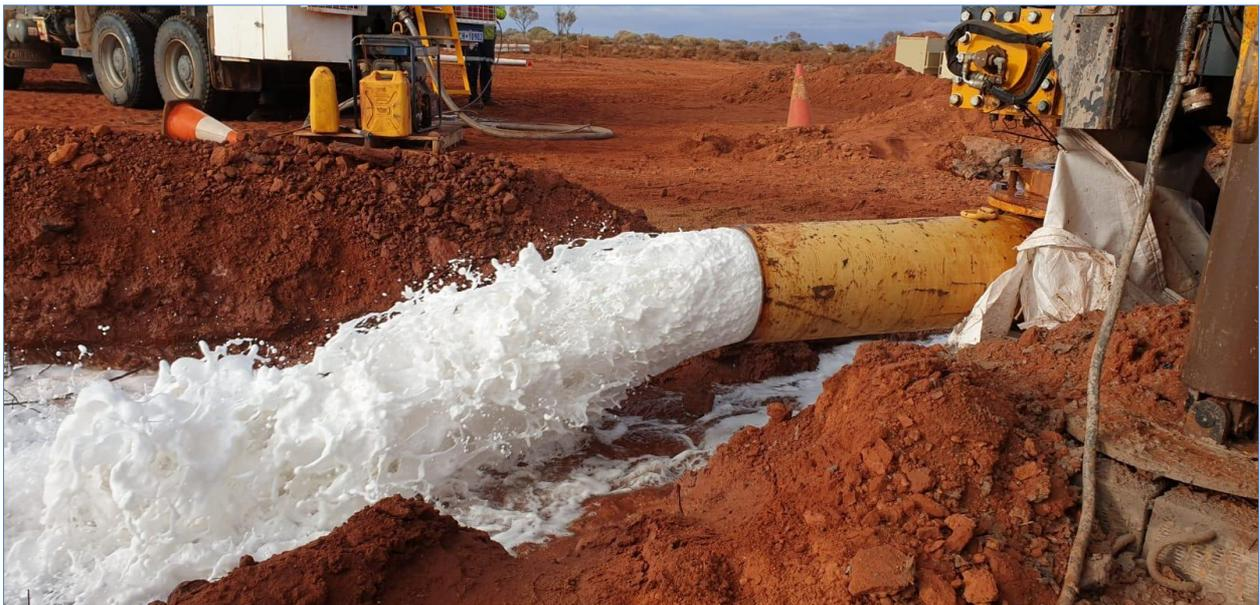
*Figure 1: 19LWPR002 being developed into the southern strike of the Lake Wells palaeochannel has been cased to a depth of 175.5m (previous deepest well cased to 170m) and is indicating very high flow rates*
