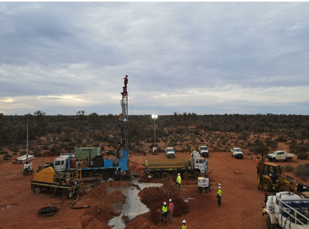
Photo 4 – Typical bore drilling setup, showing first water from the commencement of bore drilling campaign
