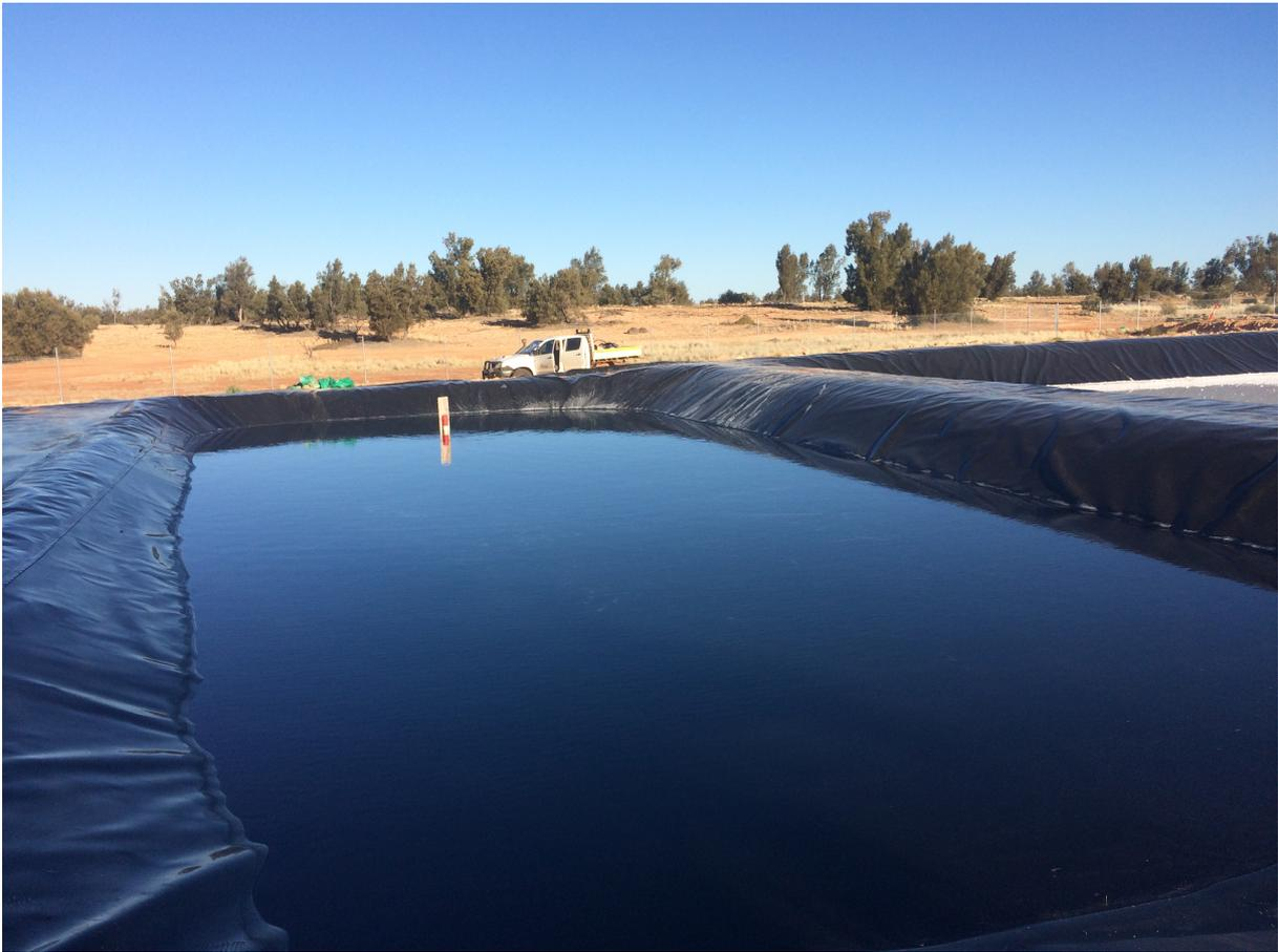
*Figure 3: Pre-concentrated brine after transfer into harvest pond 1*
