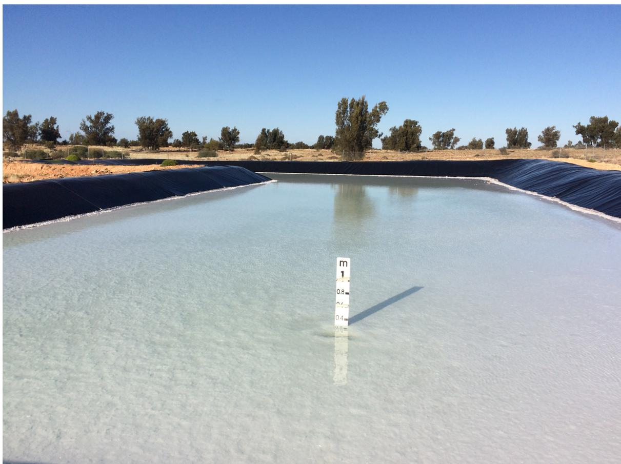
*Figure 2: Pre-concentration pond at the Lake Wells SOP project prior to initial brine transfer*
